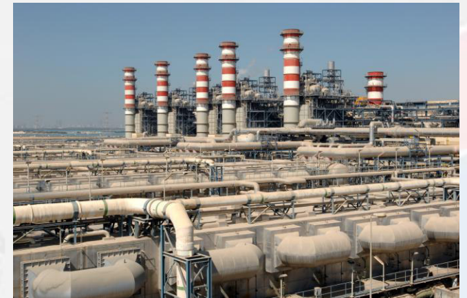
Foto (anderes Projekt) : https://www.utilities-me.com/news/article-2802-saudi-arabia-awards-siemens-590m-power-plant-deal
